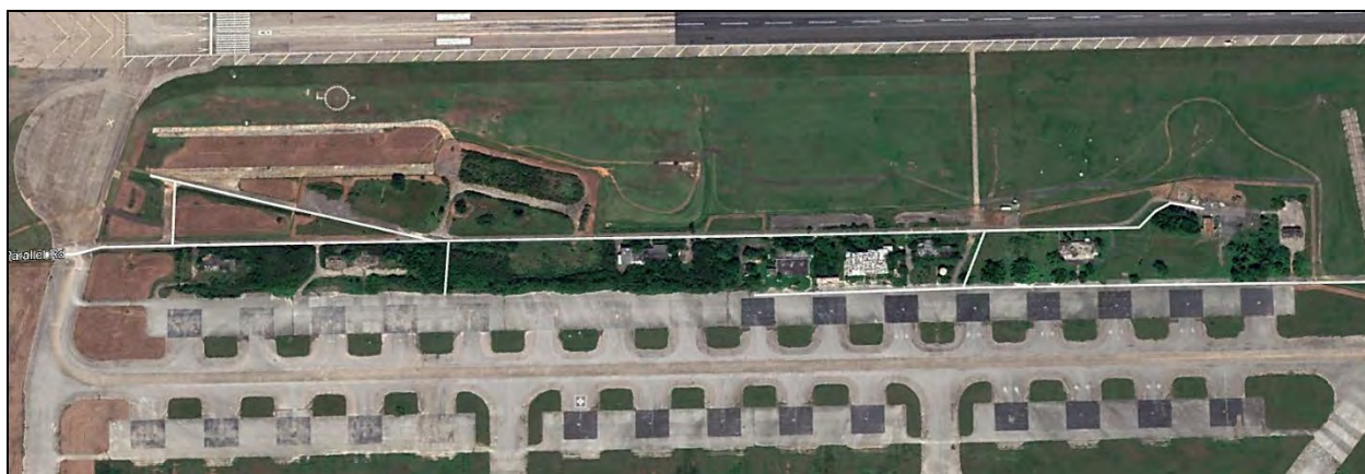
9 Photo 6.1-424 Taxiway 2 and Alert Facility apron, aerial view, 2019.
