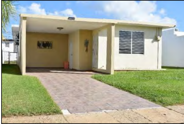
1 Photo 6.1-124 120 Loop Street
