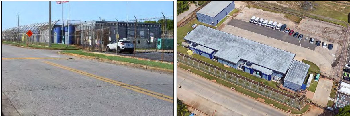
9 Building 505 (Utility Shop): Photo 6.1-195, left, south front and east side elevations; Photo 6.1-196, right, aerial view 10 depicting same elevations (source: Google Earth dated May 2016).
