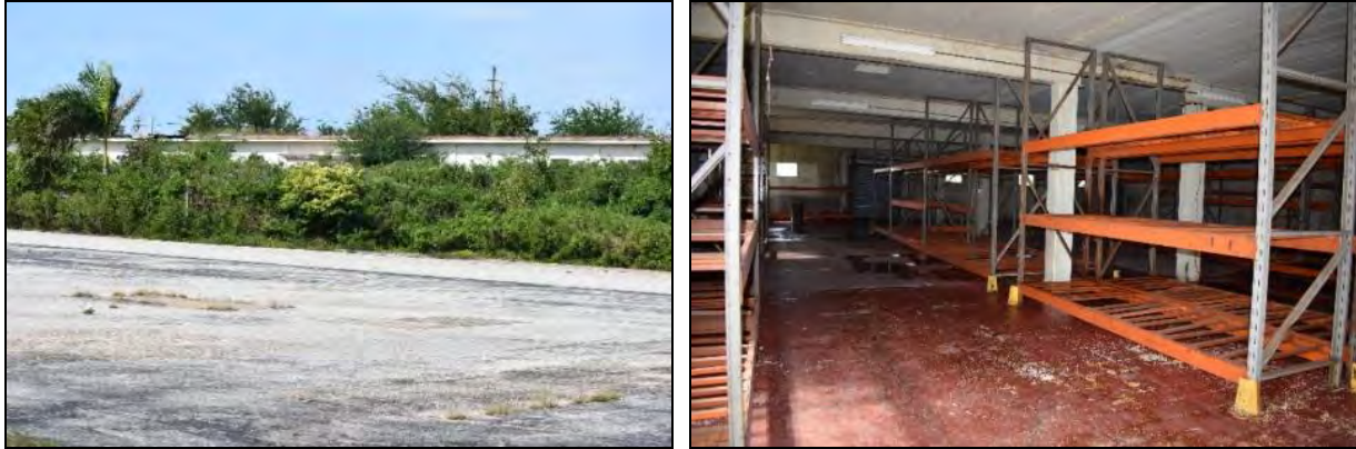
1 Building 1251 (Target Intelligence): Photo 6.1-338, left, south front elevation; Photo 6.1-339, right, interior
