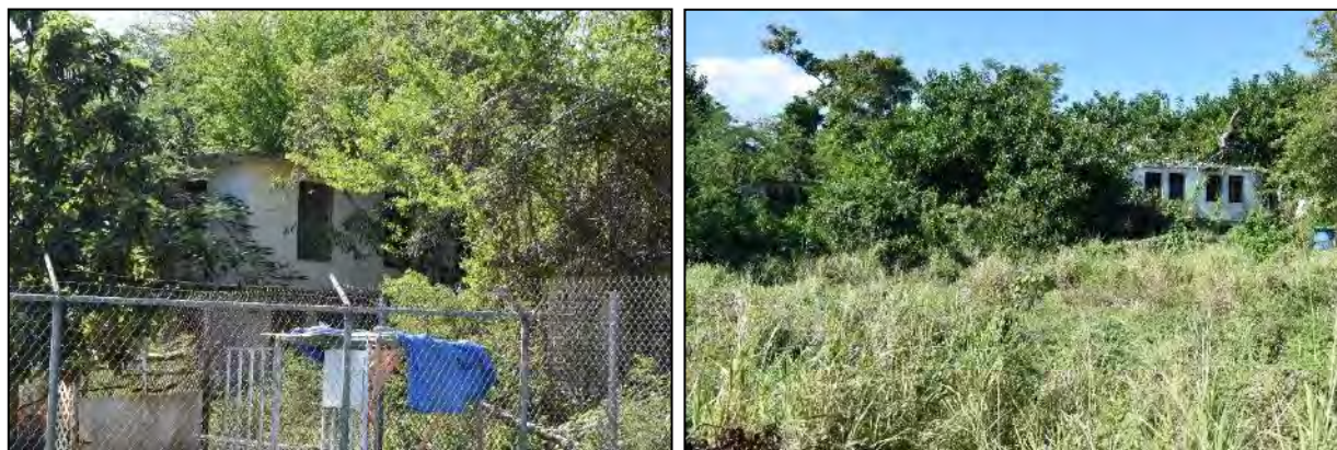
6 Photos 6.1-493 (left) and 6.1-494 (right) Current photographs looking west from PR 110R.
