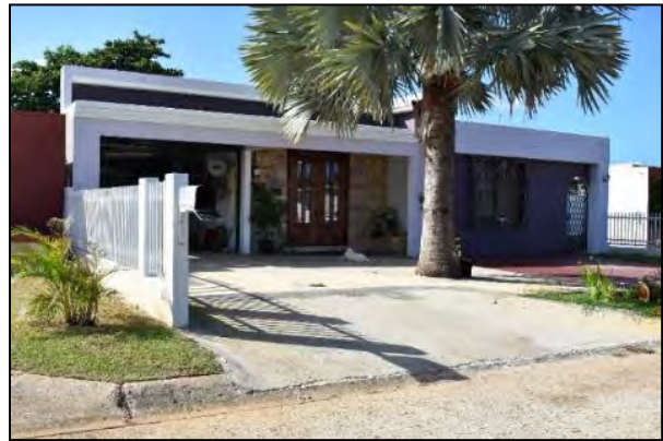
3 Photo 6.1-121 117 Loop Street
