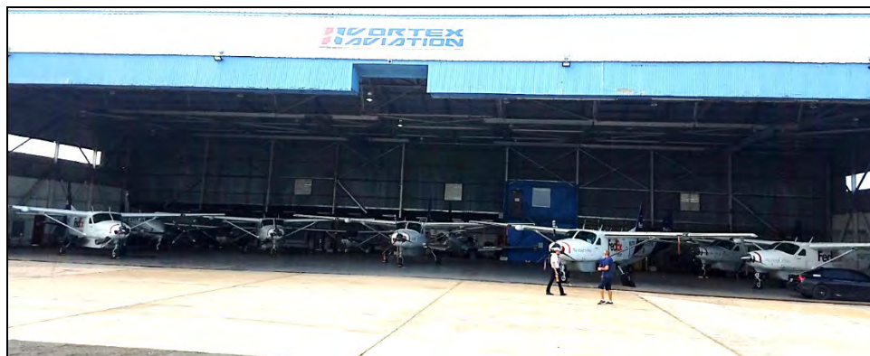
1 Photo 6.1-450 Building 573 (Nose Dock Hangar): south elevation and interior depicting retention of central notch for B- 2 52 tail, enclosure of nose dock, and addition of window bands at side elevations (source: Vortex Aviation website).
