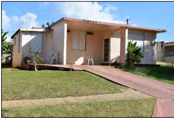
4 Photo 6.1-116 112 Loop Street
