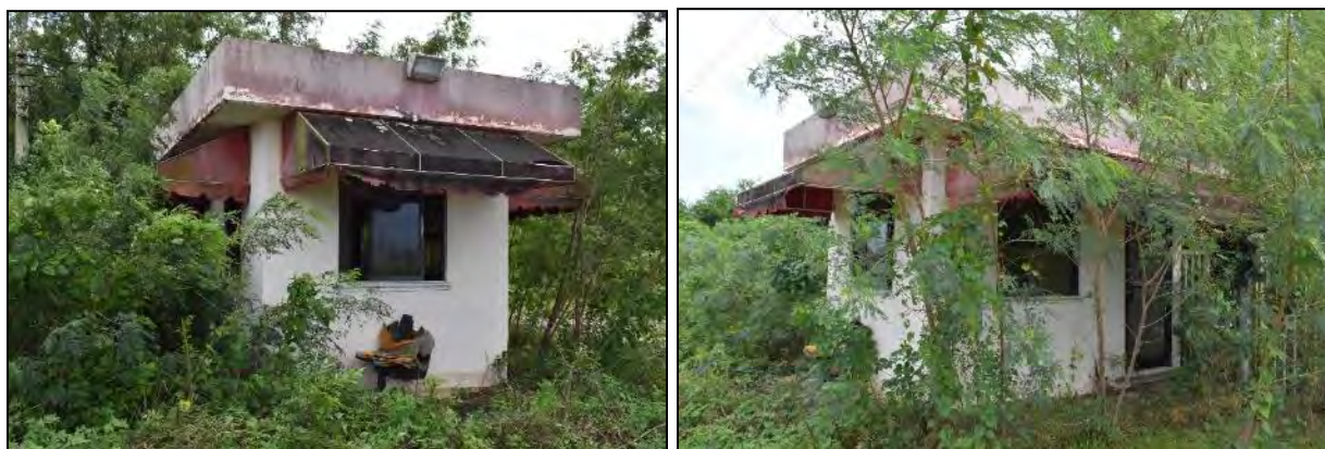
9 Guard House: Photo 6.1-362, left, west side and south front elevations; Photo 6.1-363, right, south front and east side 10 elevations
