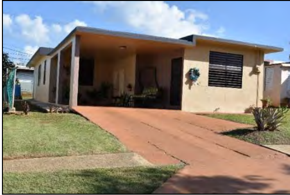
1 Photo 6.1-118 114 Loop Street
