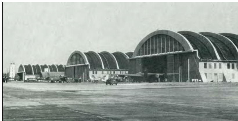
5 Photo 6.1-321 Borinquen Field, February 1944: (Left to right) Control Tower, Hangar 5, no-longer-extant building, 6 Hangar 3, and Hangar 2 (source: United States Army Air Forces, DZ Europe 1946:20).
