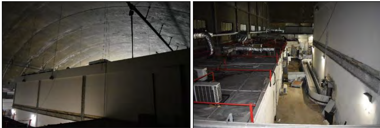
1 Hangar 5: Photo 6.1-301, left, looking south at ceiling with body of passenger and baggage claim area visible 2 freestanding on hangar floor independent of roof; Photo 6.1-302, right, another view of freestanding construction within 3 original body of hangar.
