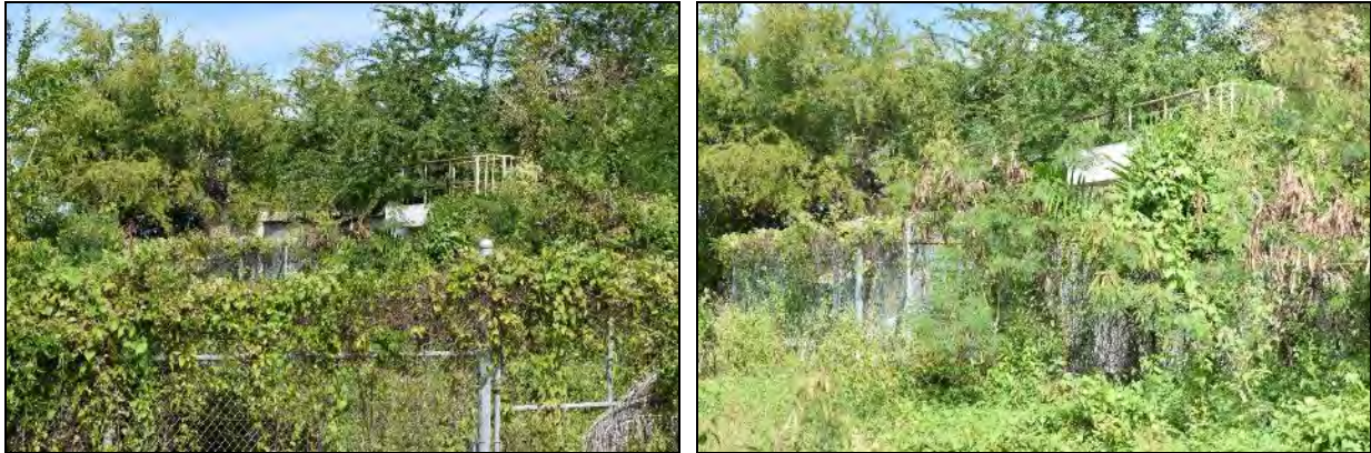
6 Water Storage Building: Photo 6.1-371, left, north elevation; west side and south front elevations; Photo 6.1-372, right, 7 north elevation framed by chain-link fencing.
