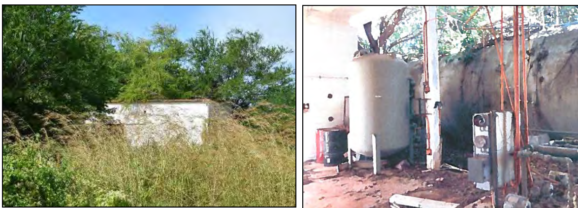
11 Building 1133 (Captive Water Supply Tank Building): Photo 6.1-369, left, south front and east side elevations; 12 Photo 6.1-370, right, interior looking northwest with large tank on right (source: AM Group 2018:98).
