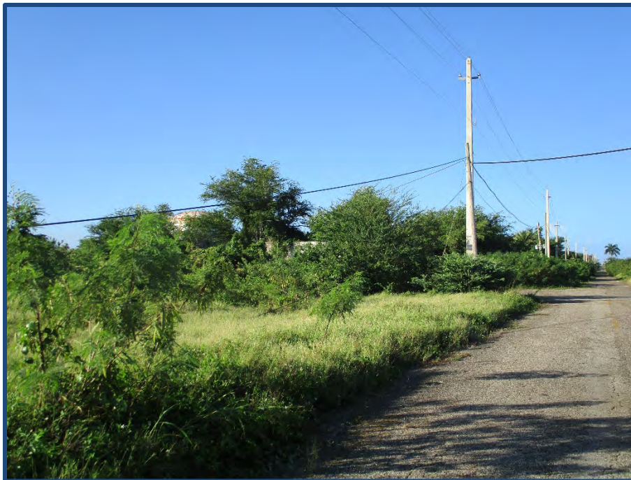
Photo 5.2-7: Overgrown locations with damaged utility risk, facing south.
