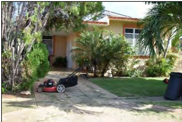
2 Photo 6.1-132 128 Loop Street
