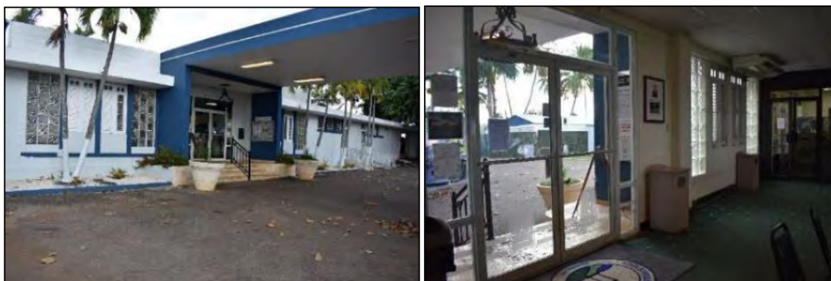
11 Photo 6.1-14, left, looking southeast at façade and later porte cochere; Photo 6.1-15, right, looking out of interior of 12 clubhouse through altered front entry and bays.
