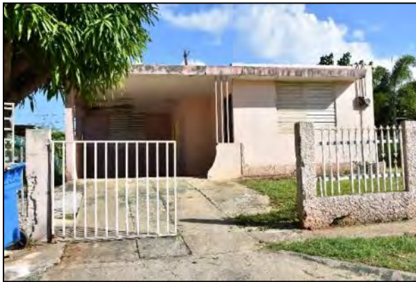
2 Photo 6.1-114 110 Loop Street
