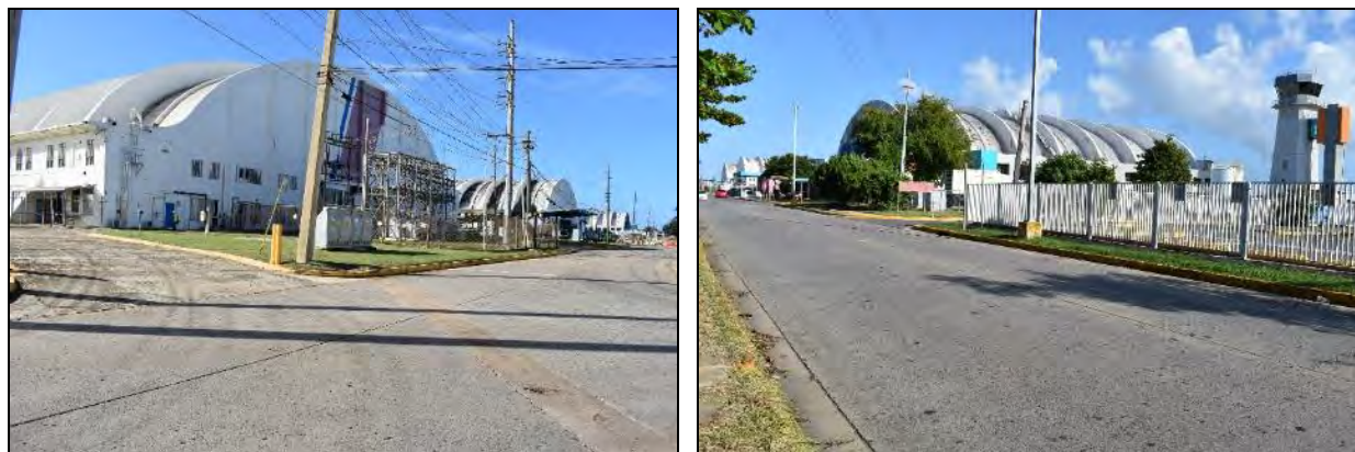
9 Photo 6.1-324, left Control Tower, Hangar 5, modern FedEx hangar, Hangar 3, and Hangar 2 (left to right); Photo 6.1- 10 325, right, Hangar 3 with Hangar 2 at far right.
