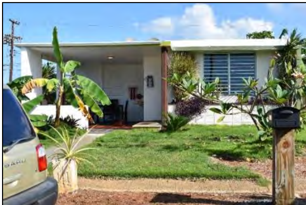
3 Photo 6.1-134 130 Loop Street
