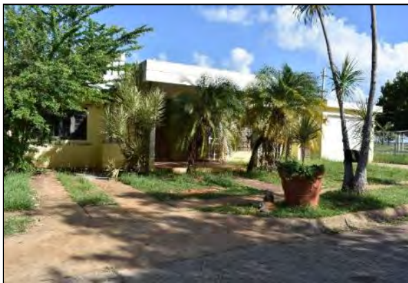
4 Photo 6.1-110 102 Loop Street
