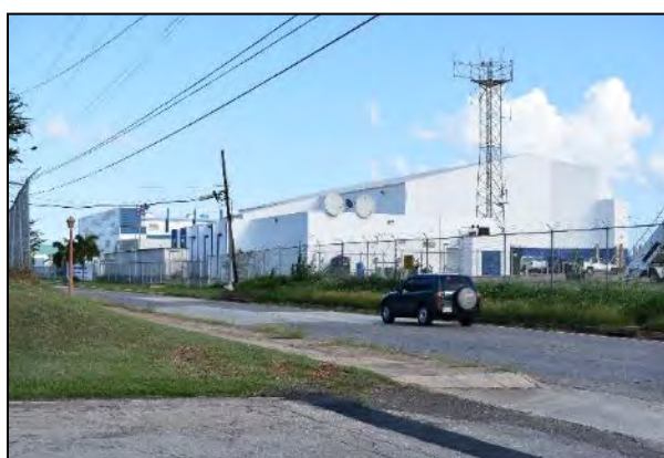
3 Photo 6.1-462 Building 575 (Hangar): north rear and west side elevations
