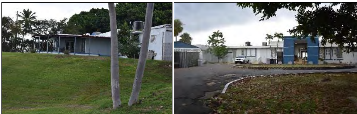
9 Photo 6.1-12, left, looking southeast at clubhouse rear with later windows, doors, and semicircular patio; 10 Photo 6.1-13, right, façade with altered bays, windows, doors, and service buildings to the west.
