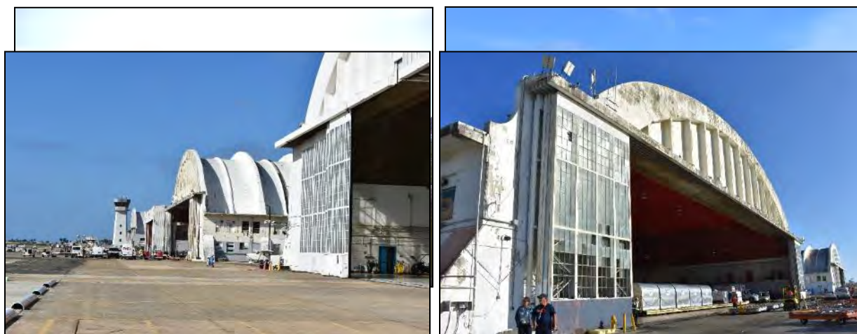
7 Photo 6.1-322, left, Views looking northeast; Photo 6.1-323, right, views looking northwest, (from left to right) Control 8 Tower, Hangar 5, modern FedEx hangar, Hangar 3, and Hangar 2.
