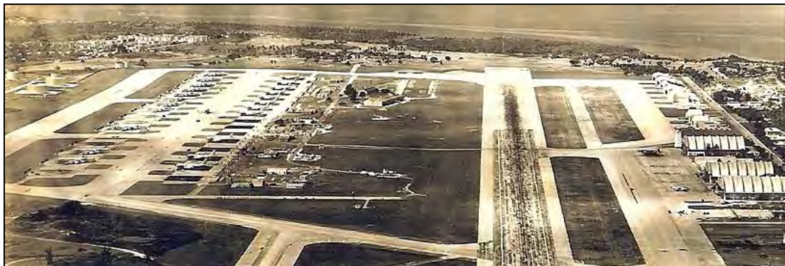
5 Photo 6.1-422 Taxiway 2 and Alert Facility Apron: looking west at taxiway and apron at left, alert facility buildings to 6 their right, and main runway at center with nose dock hangars at upper right and concrete hangars at lower right, 1966 7 (source: http://rameyafb.net/ramey-air-force-base-1966/ ).
