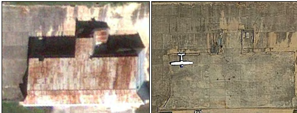
1 Building 574 (Nose Dock Hangar): Photo 6.1-455, left, aerial view in 2009; Photo 6.1-456, right, aerial view of footprint 2 in 2018
