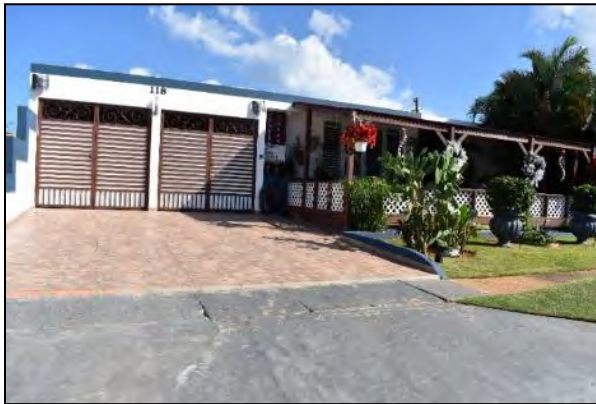
4 Photo 6.1-122 118 Loop Street
