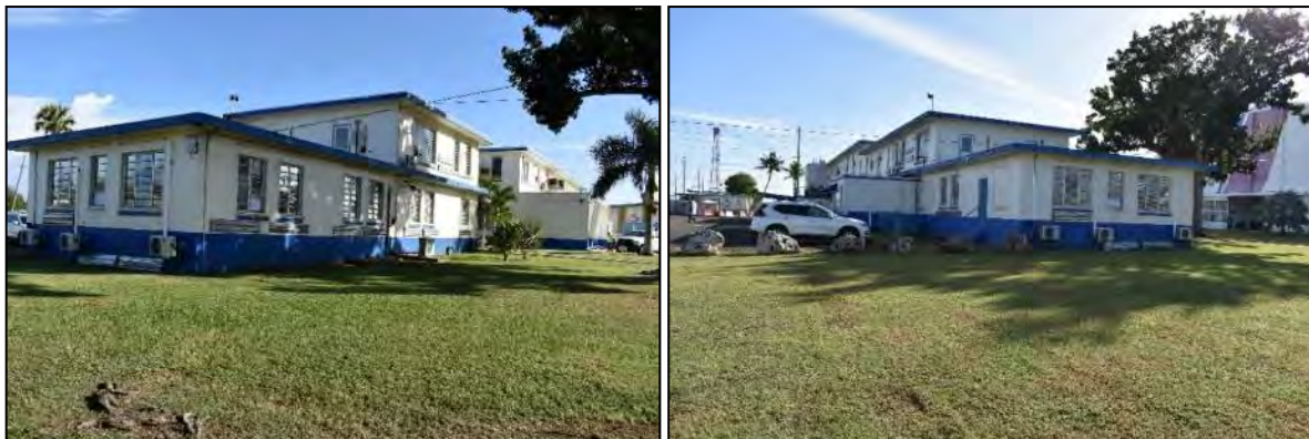
3 Building 406 (Fire Station): Photo 6.1-231, left, south front and west side elevations; Photo 6.1-232, right, west side 4 and north rear elevations.
