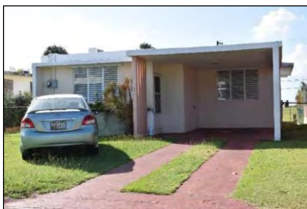
Photo 6.1-26 Largely intact houses: 125 Loop Street
