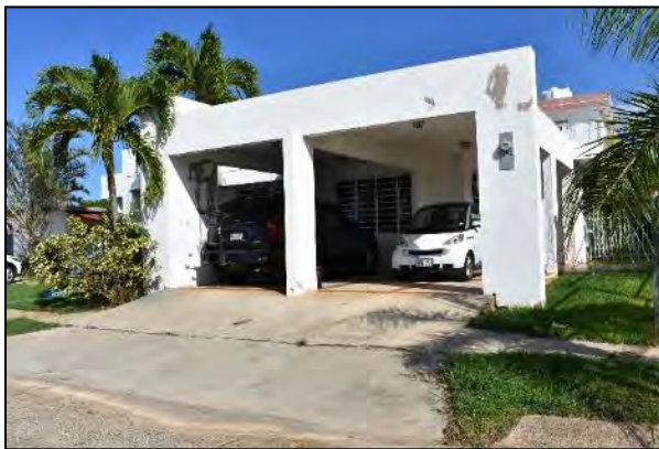
4 Photo 6.1-128 124 Loop Street
