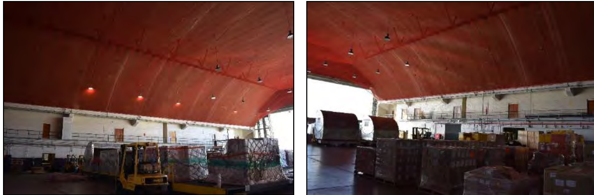
1 Hangar 3: Photo 6.1-288, left, looking southeast toward east flank of rooms and runway-side elevation; Photo 6.1-289, 2 right, looking southwest toward west flank of rooms and runway-side elevation.
