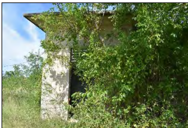
13 Photo 6.1-335 Building 1270 (Storage): S front elevation.
