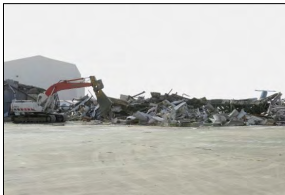
3 Photo 6.1-457, Building 574 (Nose Dock Hangar): hangar demolition (source: RAFBHA 2015e).
