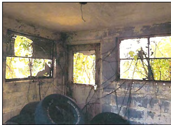
11 Photo 6.1-421 Building 1073 (Traffic Check House): interior (source: AM Group 2018:150)
