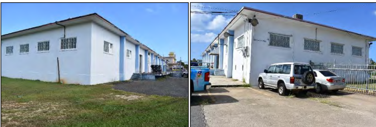
7 Building 503 (Quartermaster Warehouse): Photo 6.1-189, left, west side and south rear elevations; Photo 6.1-190, right, 8 south rear and east elevations.
