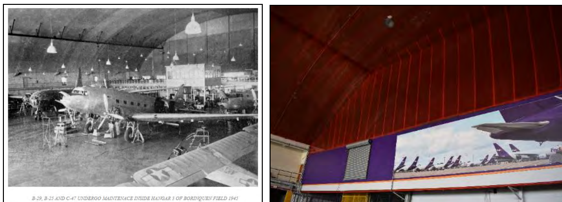
14 Hangar 3: Photo 6.1-286, left, looking northwest at hangar interior in 1945 (source: RAFBHA 2015b); Photo 6.1-287, 15 right, looking northwest at north wall and roof; note that wall, roof, and hanging light supports beneath mesh continue 16 to look those in the 1945 image.
